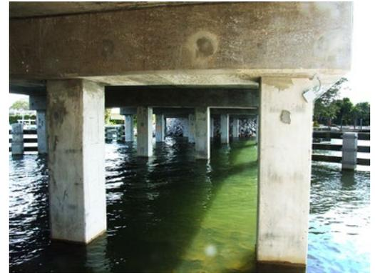
*Precast piles fit into grouted sockets in the horizontal precast bent cap which supports the bridge deck.*
